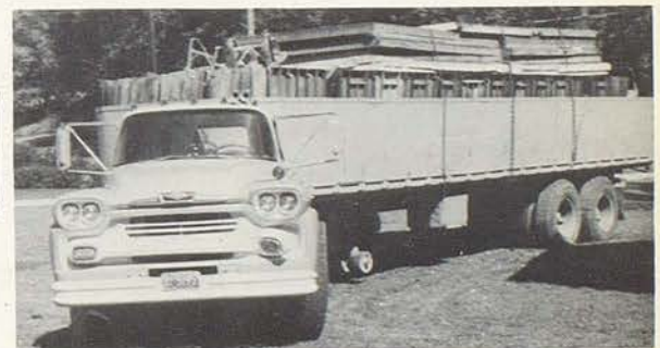
The first load arrives for the new construction
