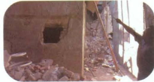
An earthquake measuring 7.8 magnitude rocks Colima, Mexico. Iran and Italy experienced major quakes measuring 6.3 and 5.9.
