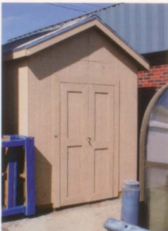
Above: The building trades class constructed an equipment shed between the crow's nest and ag shop. Photo by Steven Clary
