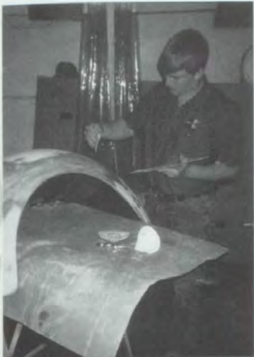
Adam Stevens applies putty to a project he is working on for Auto Collision Repair.
