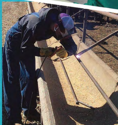
Carter Jensen welds a piece to prevent cattle from getting through a cattle feed bunk for his demonstration of knowledge hours.
